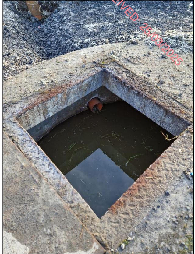
PHOTO 2. SEPTIC TANK OUTLET
