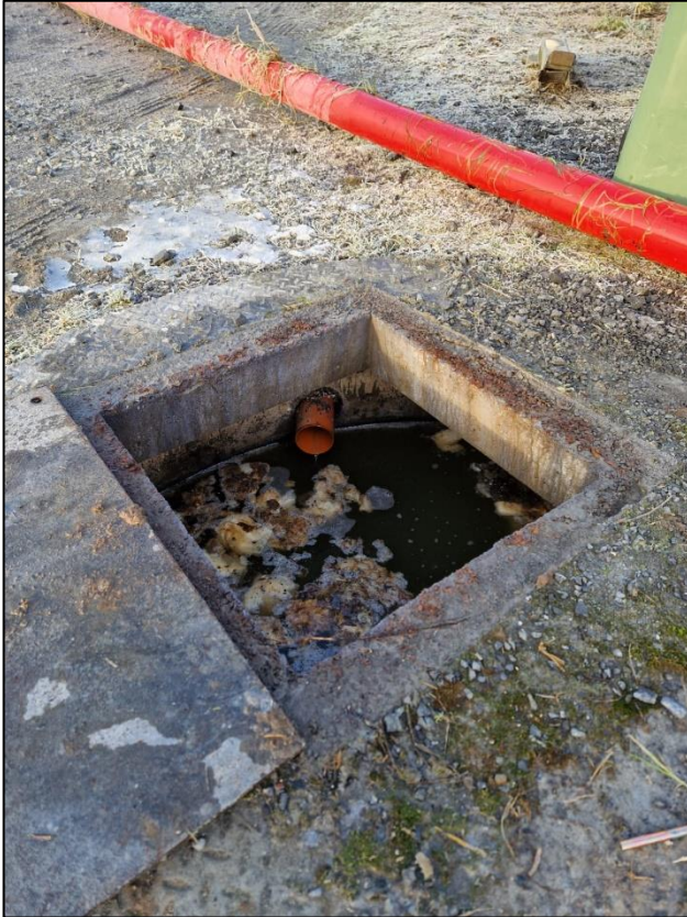
PHOTO 1. SEPTIC TANK INLET
