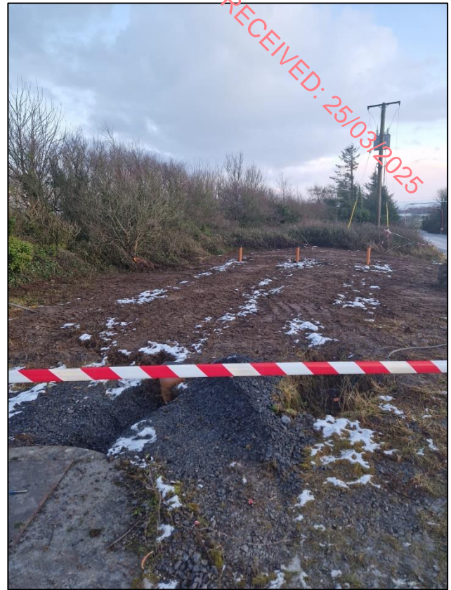
PHOTO 5. PERCOLATION AREA, WITH VENTS VISIBLE AT THE ENDS
