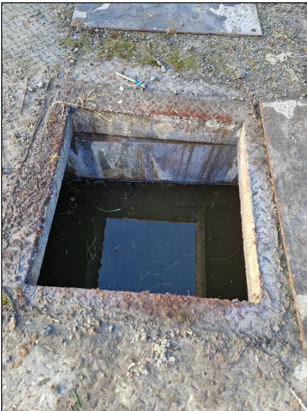
PHOTO 3. BAFFLE WALL
