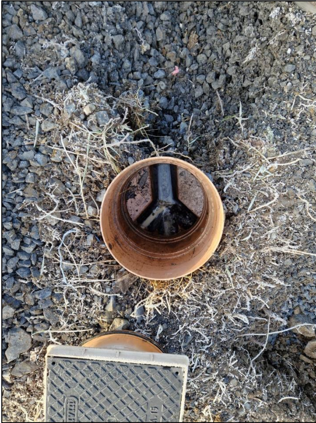
PHOTO 4. DISTRIBUTION ACCESS JUNCTION
